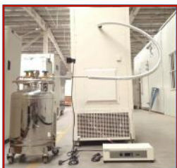
LN 2 /CO 2 backup system
